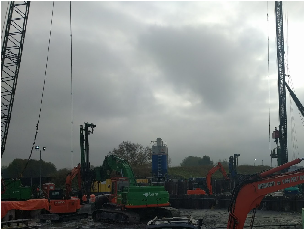
Figure 6. The South Tunnel Approach during foundation construction
